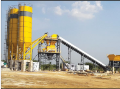
CONCRETE BATCH MIX PLANT
